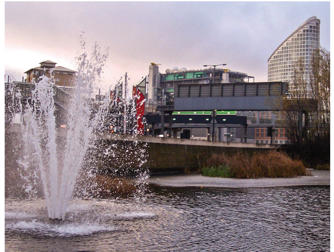
The East India Dock Fountain splashed passing cars until Wilson Electric Engineers solved the problem.
