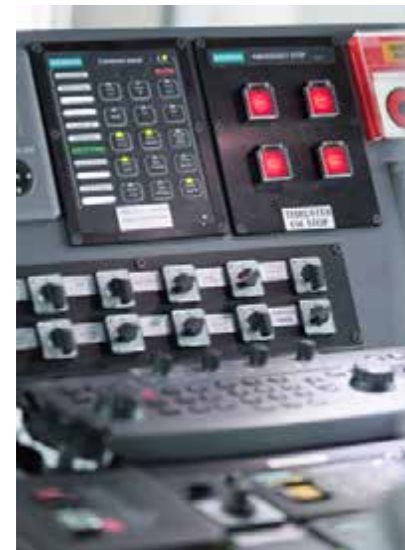
The ship's genset, switchboard, propulsion and thruster control systems are fully integrated to ensure seamless ship operation.
