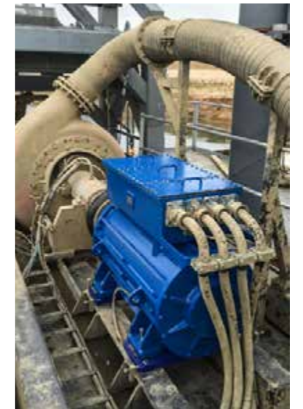
Submersible motor cleaned after testing & Commissioning.
