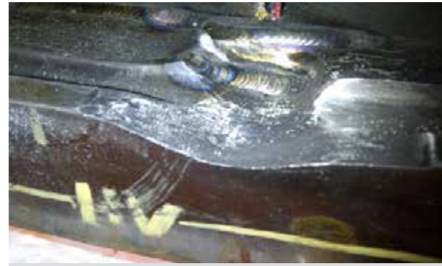
Figure 20. Slot 11 ready for weld repair.
