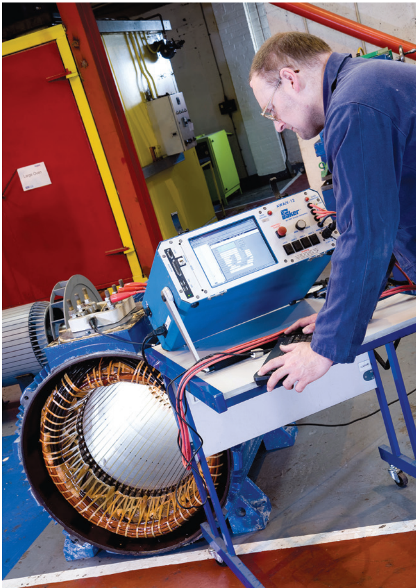
Testing a motor after rewind at Team Rewinds
