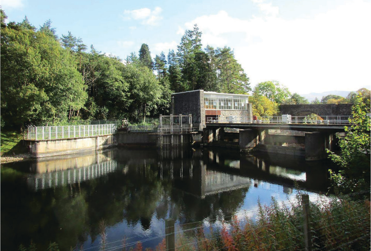
Quartzelec completes bespoke brushless exciter retrofit at Mucomir Hydro
