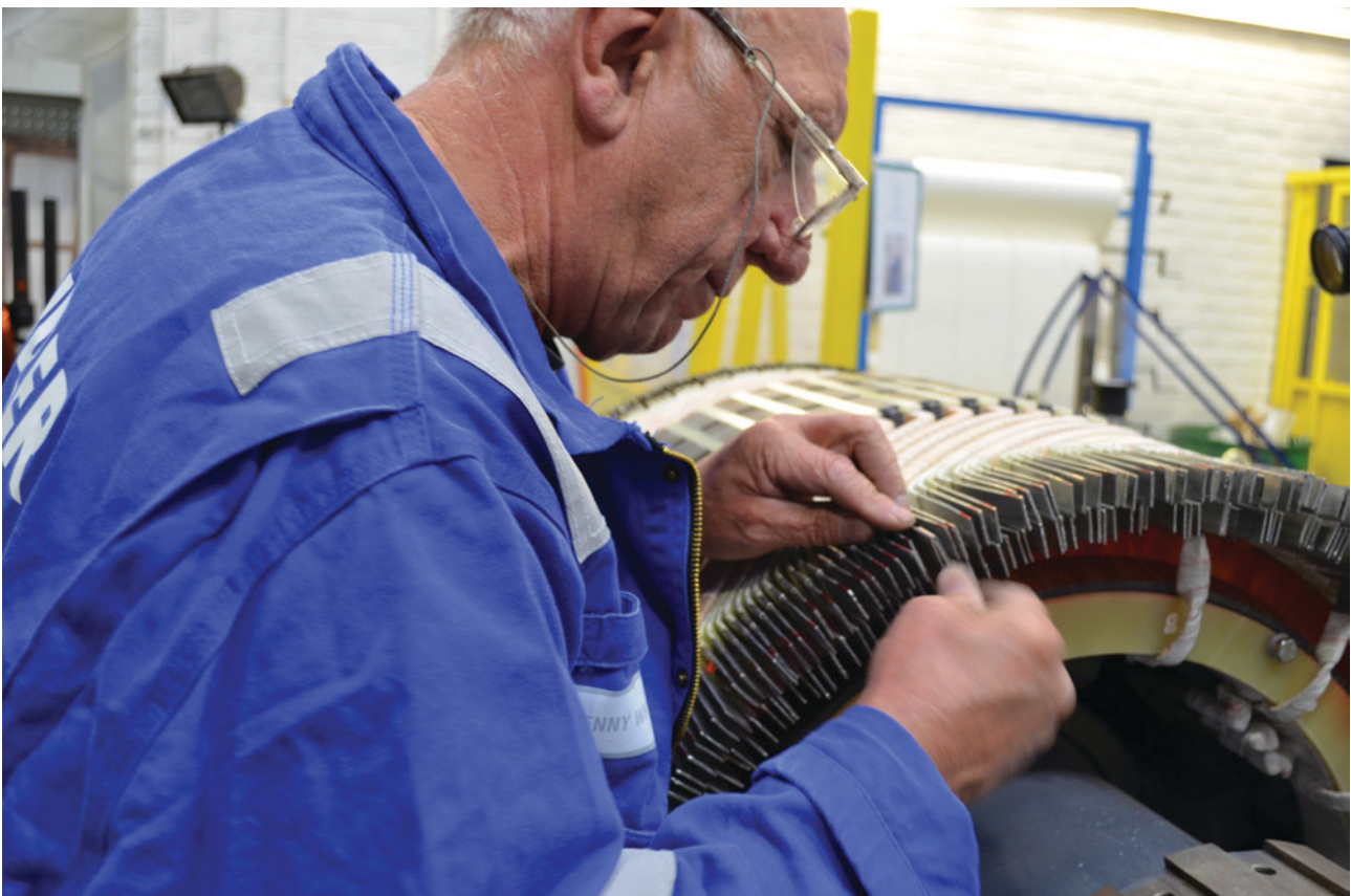
The damaged components were rewound while the investigation into the cause progressed
