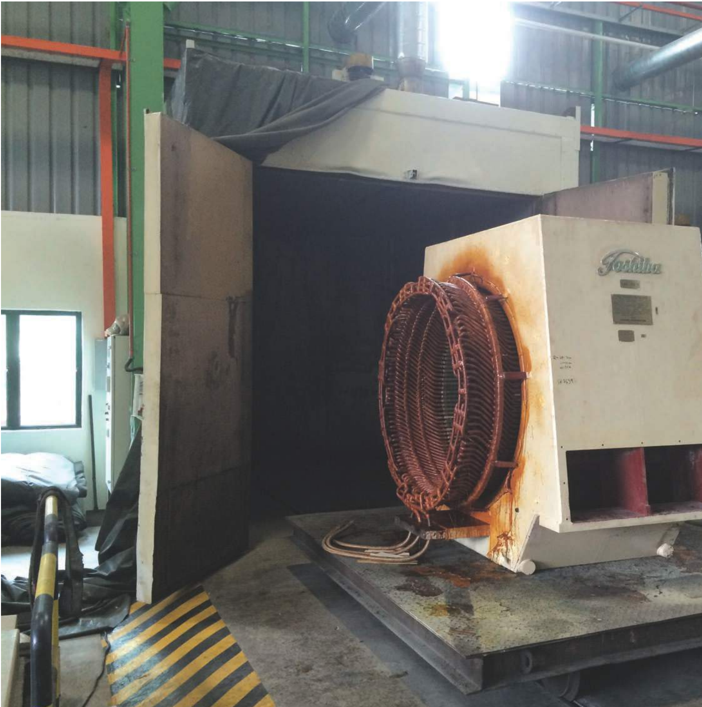
The oven at Siemens Malaysia used for 2250kW Stator after rewinding.
