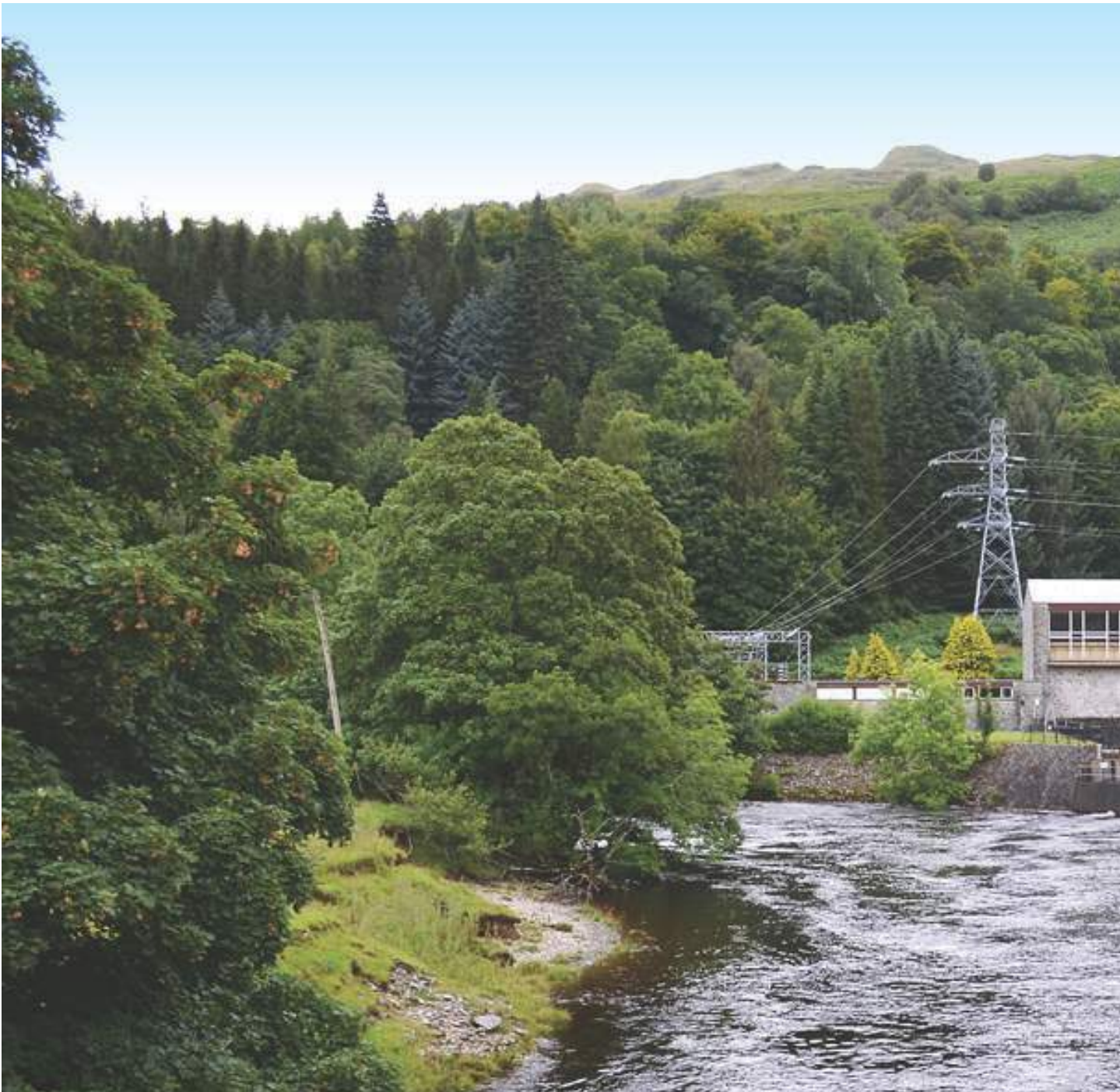
After nearly 60 years of service the hydro generator at Lochay Power Station was scheduled for refurbishment and the project was awarded to Sulzer, which has a distinguished history in high voltage generator refurbishment.
