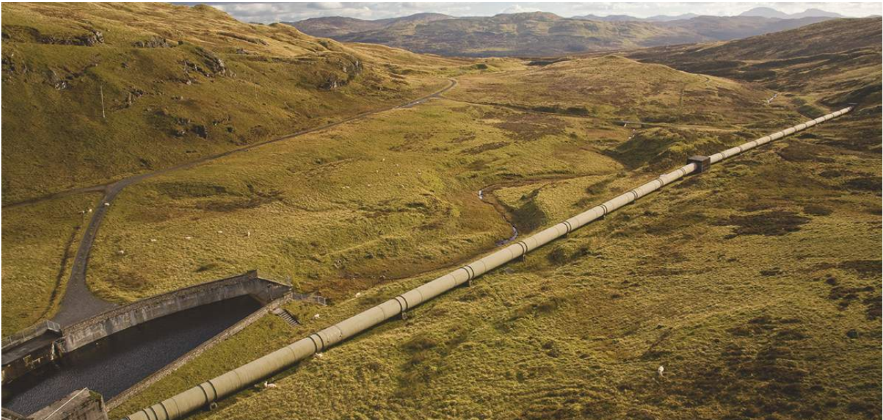
The Breadalbane Hydro-Electric Scheme is located in the mountainous region in highland Perthshire and utilizes the water stored behind 6 dams. Over 20 tunnels and aqueducts carry water to 7 power stations, of which Lochay Power Station is the largest.
