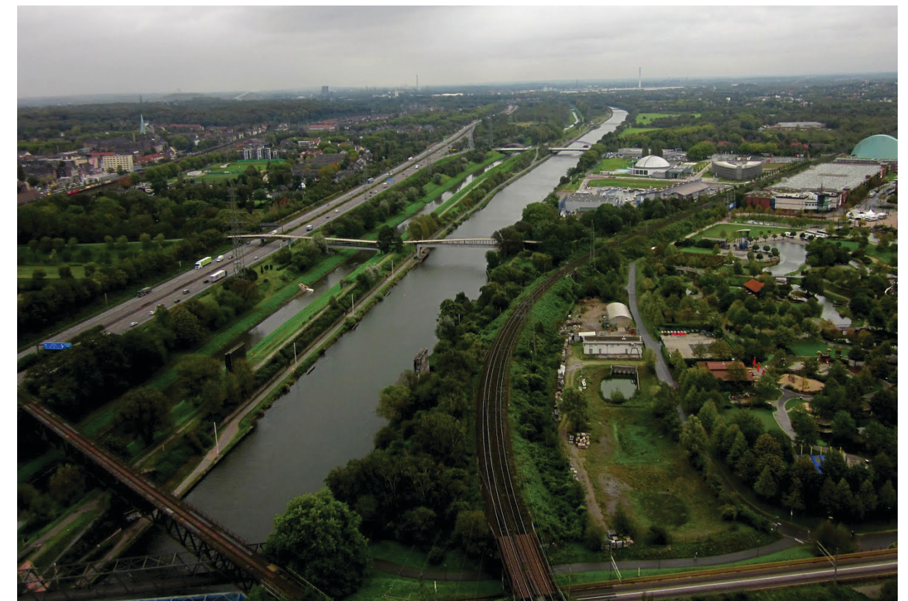
Pump failure could have a catastrophic impact to the canal side environment.
